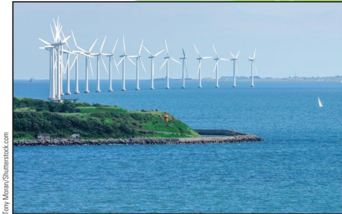
Figure 10.24: Danish offshore wind farm.
