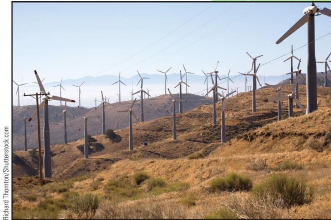
Figure 10.22: Tehachapi wind farm in California.
