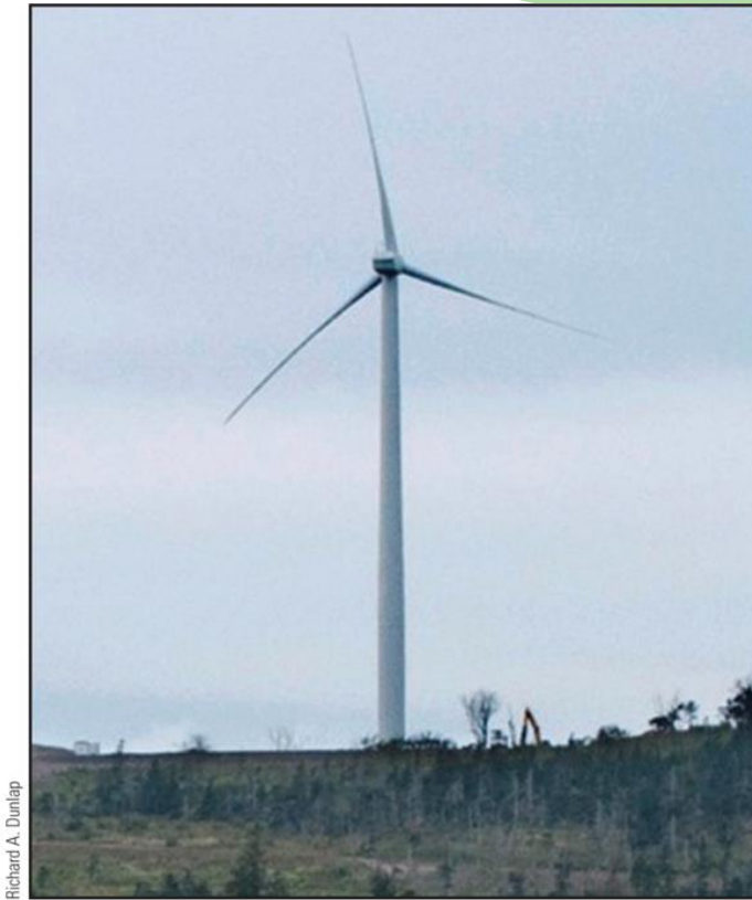
Figure 10.6: Modern three-blade wind turbine at Digby Neck Wind Farm, Nova Scotia. Turbine is a 1.5-MW GE 1.5sle with a rotor diameter of 77 m and a hub height of 80 m.
